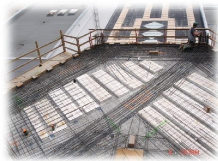
Figure 11: Filigree Construction Photo
